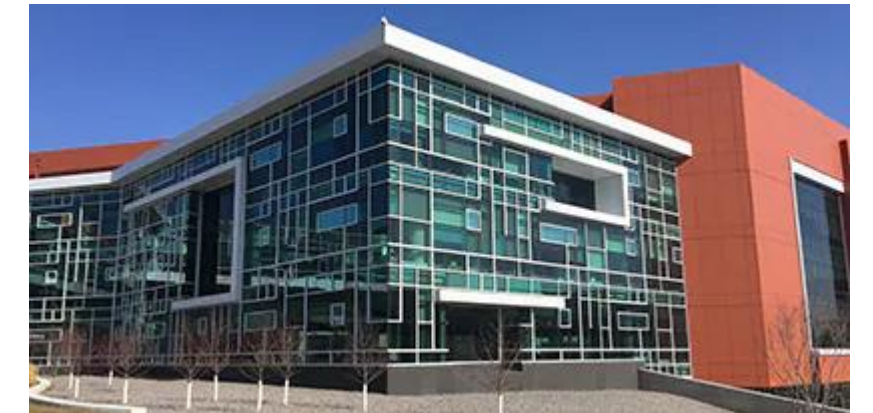
Construction (glazing, multimaterial panels)
